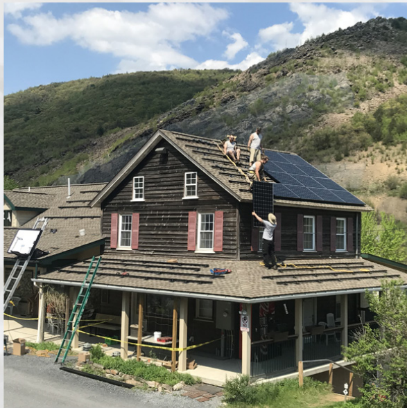
Solar Panel Installation 2018
