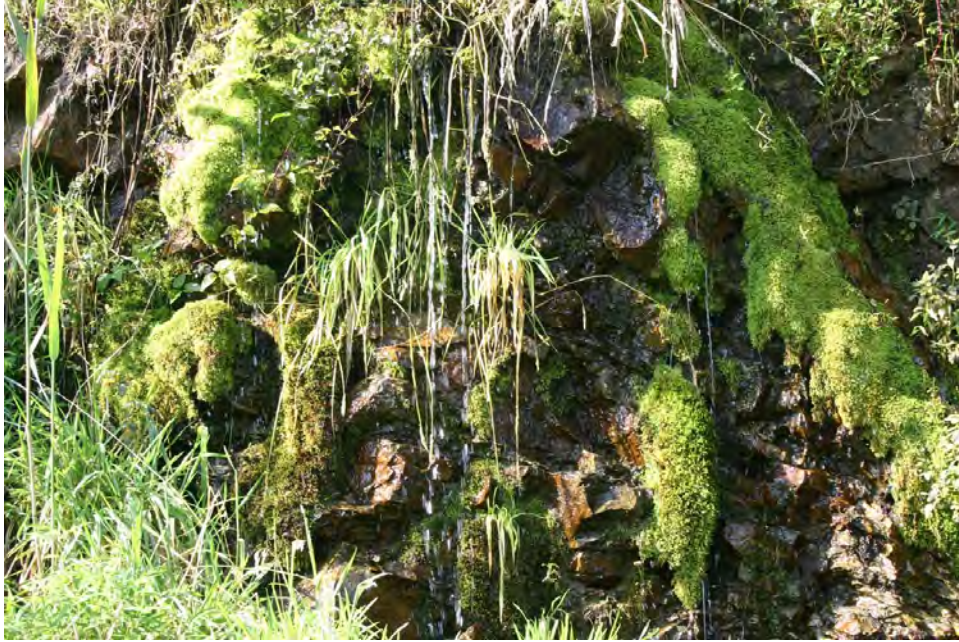
A Seep along the D&L Trail
